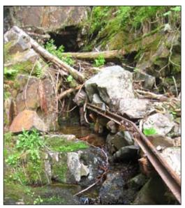
The collapsing adit of the Regal Mine and rusting rails are left from the prospecting era
